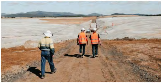
Surf Lakes nears completion.
